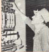
Walter Bullard's Electrician in the Steel Shop (Night). He began work here in July, 1942, having worked last previously in a Hydro-Electric Plant in La Grange County. Walter is married and has two boys. He says that his outside interests are not many, but Pat Photography enjoys working in his garden and yard at all times.
